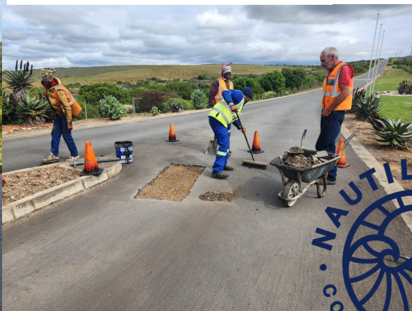
Trukon team on site.
