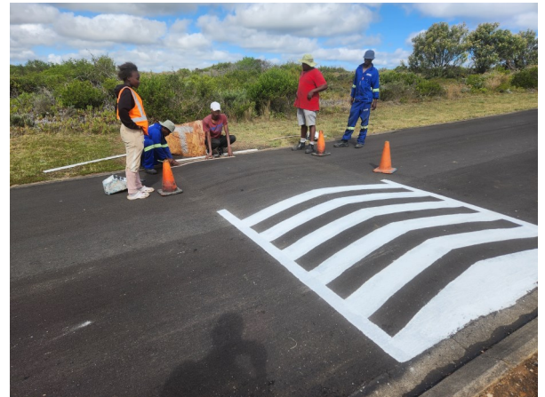
Trukon busy with final touches
