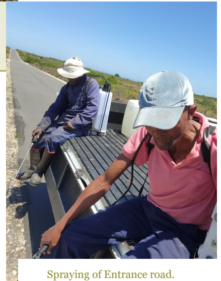
Maintenance at the reservoir
