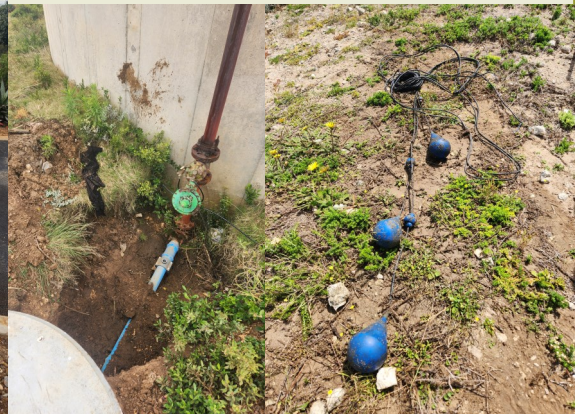
Repairs at the Reservoir
