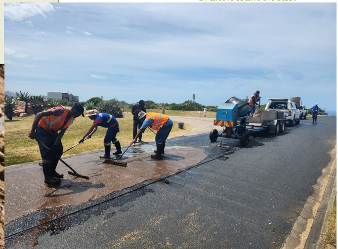
Trukon team on site.
