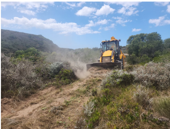
TLB on-site improving road accessibility.
