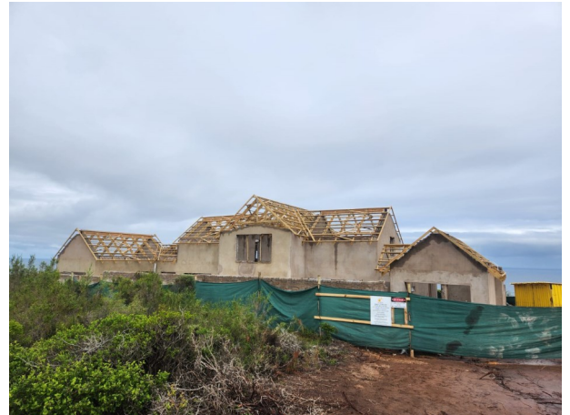
Unit 32 under construction.
