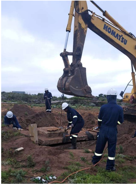
PetroSA completed work
